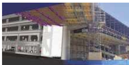
LINXS Constructors selected BrandSafway to provide access to the underside of the automated people mover (APM), the APM stations and walkways during construction at LAX.
