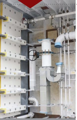
A completed block demonstrates the need to coordinate workflow between insulation installers and the mechanical, electrical and welding trades
