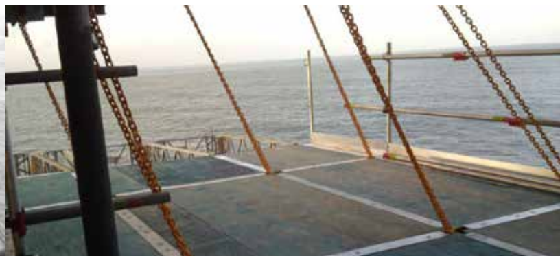
QuikDeck delivered a safe, smooth surface to paint the entire offshore natural gas platform.
