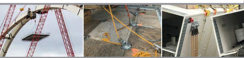
With capacities up to 150 pounds per square foot, built from a few basic modular components and outfitted with guard rails
