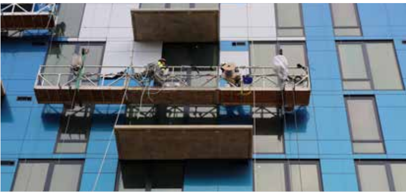
Skilled trades that used the swing stage platform also included those installing window caulking. ⤴
