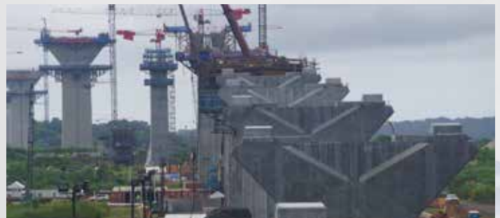
Panama Canal Bridge, Panama | Pier and bridge construction | Aluma Systems® forming and shoring
