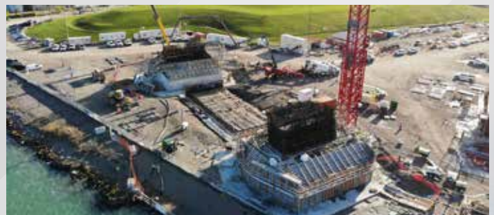
Gordie Howe International Bridge, Canada and USA | Forming and access for new bridge construction | Formwork, falsework, stair towers, access platforms, elevators and engineering
