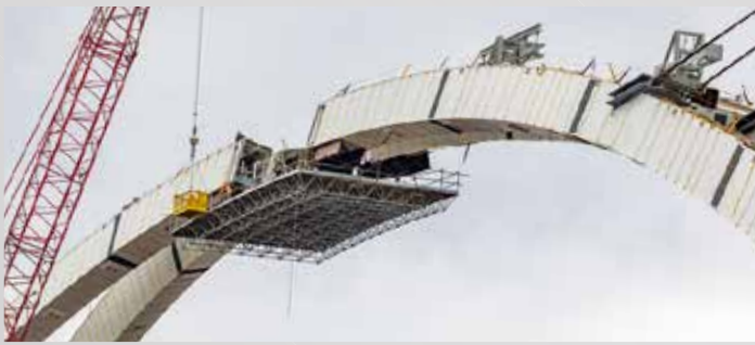
I74 Bridge, Illinois and Iowa | Keystone placement in arch | Truss Frame System, rotating suspension point (RSP) brackets, engineering
