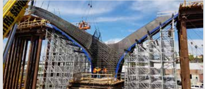
Sixth Street Viaduct, California | New build | Aluma Systems® custom formwork and heavy duty GASS™ shoring
