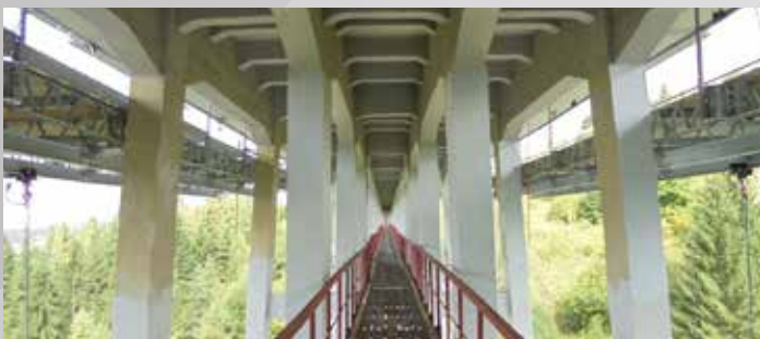
Caracau Viaduct, Romania | Rehabilitation of 264-meter railway bridge | Rope access, QuikDeck® Suspended Access System, rotating suspension point assemblies, steel monorails and swing stages
