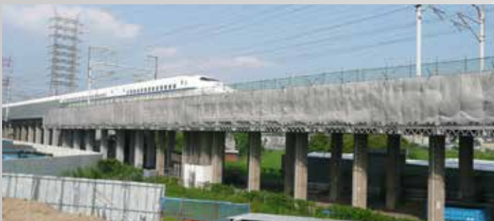
Shinkansen Railway Project, Japan | Retrofitting 90 miles of elevated track | QuikDeck® Suspended Access System
