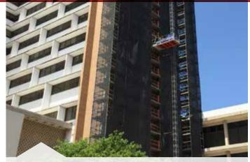
Move large loads up to 12 feet in length. Designated operator not required. VFD (Variable Frequency Drive) technology ensures a smoother, quieter ride.
