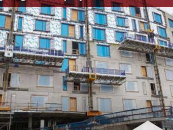
Ability to expand upper work area and install a low floor on outriggers to create ideal work environment.
