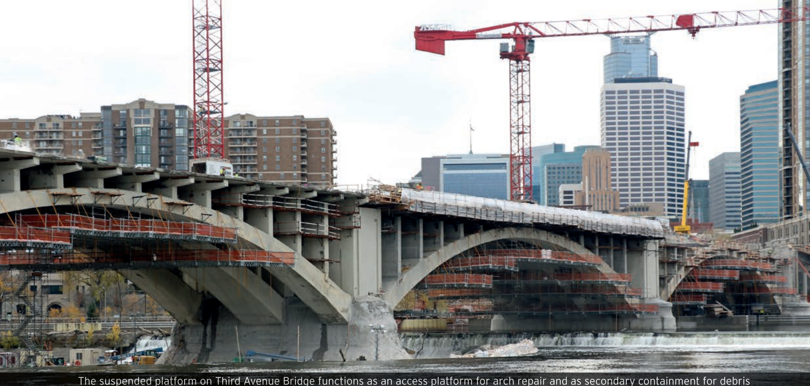
The suspended platform on Third Avenue Bridge functions as an access platform for arch repair and as secondary containment for debris
