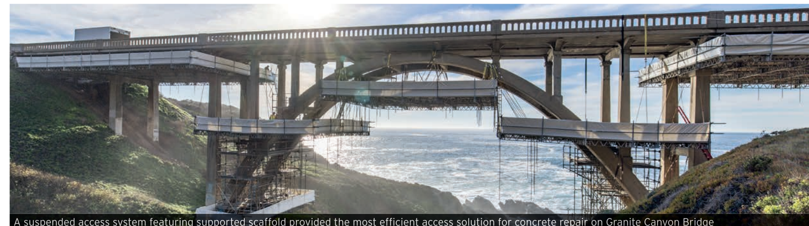
A suspended access system featuring supported scaffold provided the most efficient access solution for concrete repair on Granite Canyon Bridge
